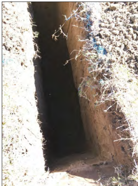
View looking at Pit 4 excavation. Note collapse (undercutting) of right wall.
